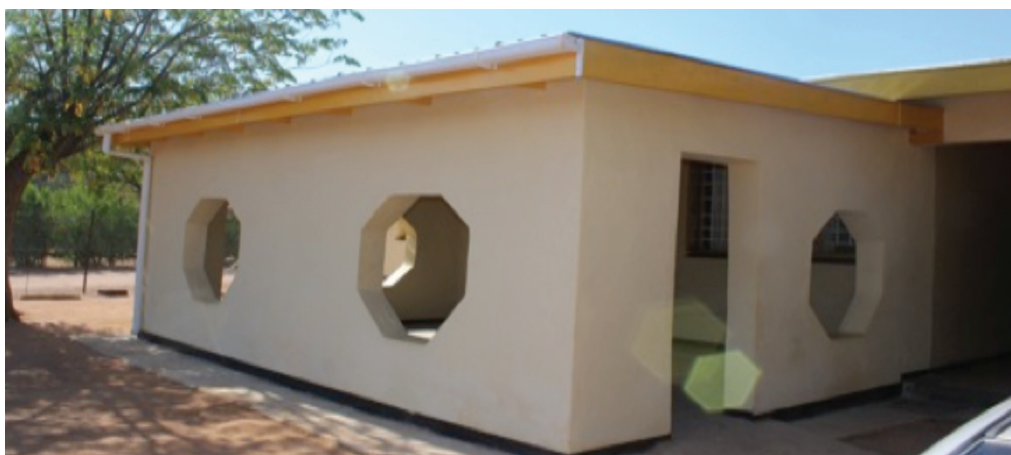
The new waiting area at Mochudi Clinic 1, built with community funds
